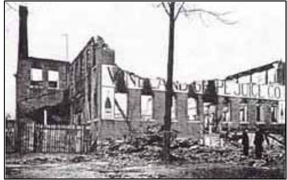
Aftermath of a fire that destroyed Vineland Grape Juice Company in 1913.
