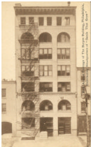
The W.A. Burpee Building
